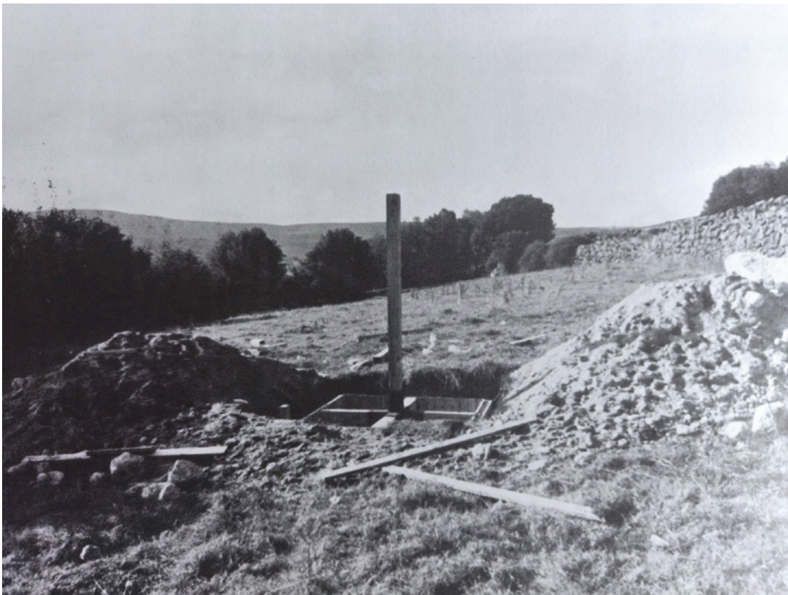
Excavation of Cloon, Spring 1980. Photo by Brian King.
